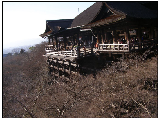
Kiyomizu Temple Foundations Built without Nails
